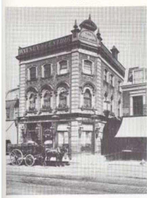
The former Black Horse pub in Brixton Road – closed c.1966 and the upper part later used as offices by the Central Lambeth Project.
