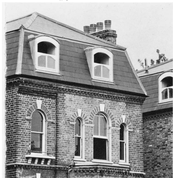
Houses on the north side of Loughborough Road newly-refurbished by Lambeth Council c. 1978. Bx-LR2.jpg, courtesy Marley-Eternit
