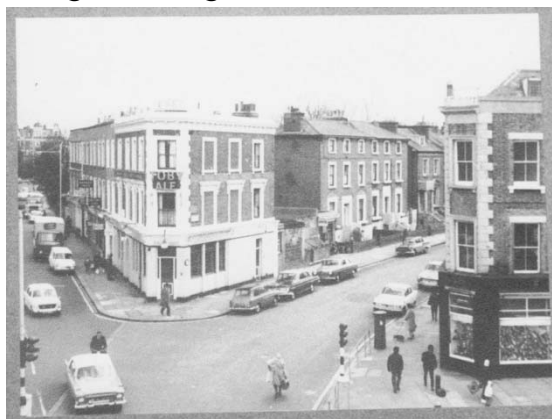
Looking into Loughborough Road from Brixton Road c. 1966, with Angell Road running diagonally to the right - all demolished to make way for building the Angell Town Estate in 1974-76. Bx-LR1.jpg
