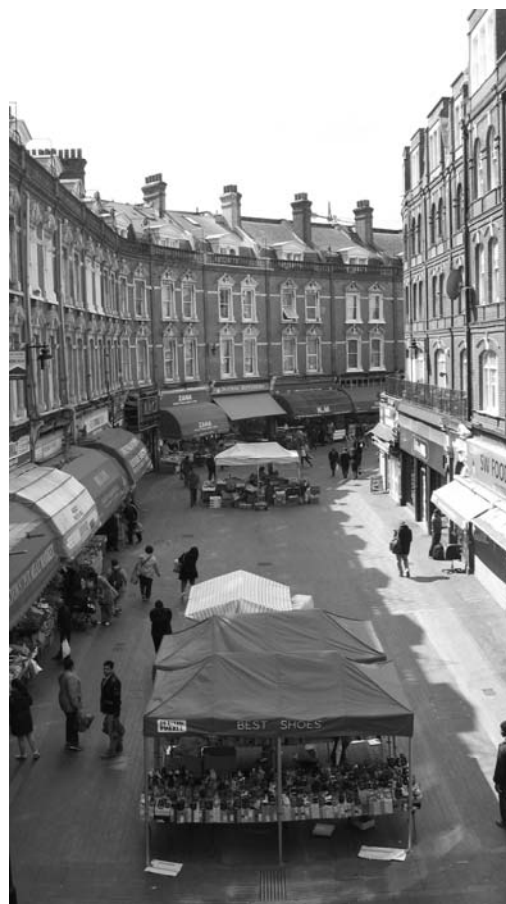
Electric Avenue after completion of the repaving works (Bx&R17-07.jpg)
