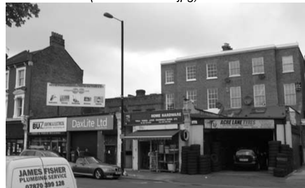
Changing trading patterns on Acre Lane: 90-92 were built as houses in the 1830s, with shops built over the front gardens in 1884 (2013 photo). C832-My13-10.jpg
