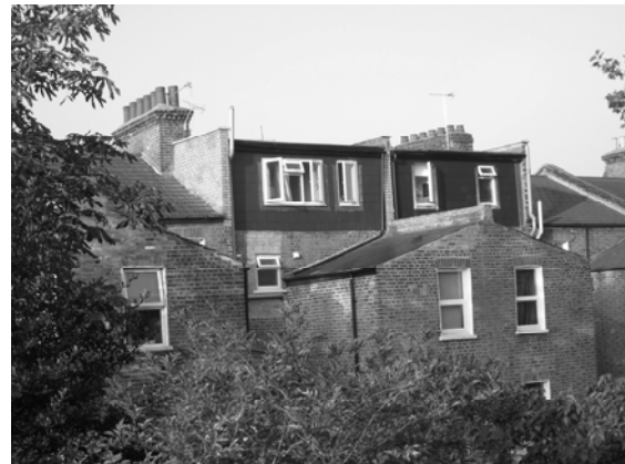
Roof extensions in Railton Road.
