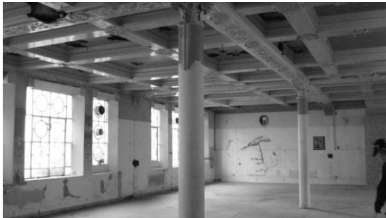
Upper floor office space before refurbishment, May 2015 (BTC-tpin15-04.jpg)
