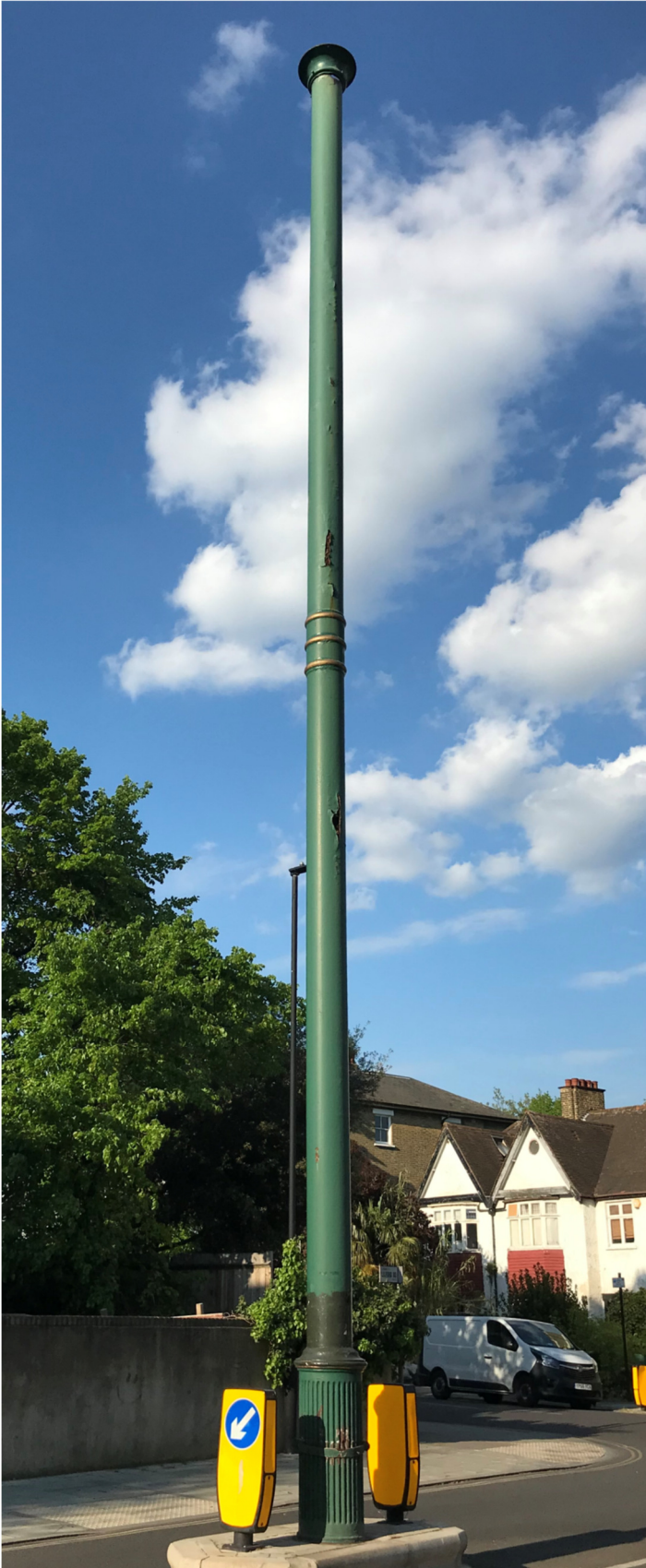
The original pipe
