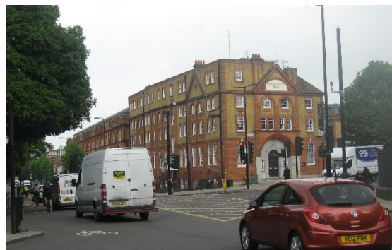
1-3 Brixton Road, showing frontage to Camberwell New Road (Db/CU-2018-06-01-02.jpg)
